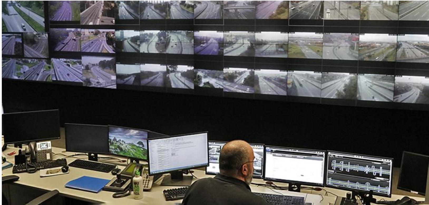
**TT3. Road Traffic Control Centre**, enabling participants to acknowledge a road administration control centre, where road traffic is monitored in real time and support to traffic flow and user assistance is provided.
